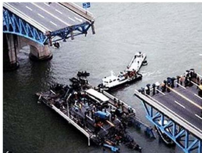
Fig.2: Collapsed Steel bridge - Seongsu Bridge, Korea, 1994 (Wang et al., 2017:51).
