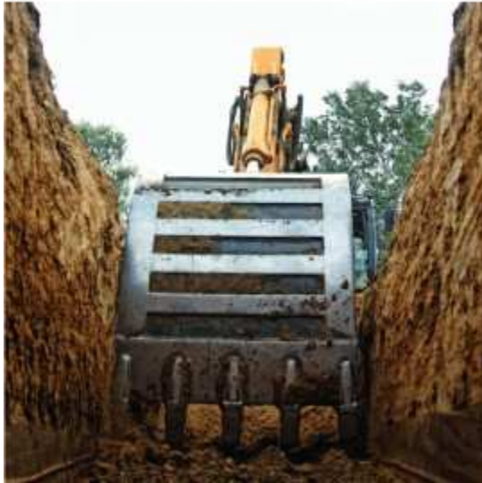
Figure 2: Excavation works with an excavator Source: Gurley, 2012).
