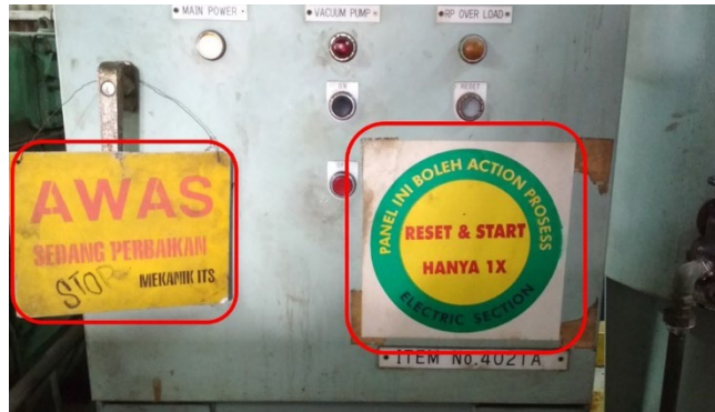
Figure 2 Tags that function like red tags on the vacuum pump in the spinning area. (Source: PT ITS, 2018)
