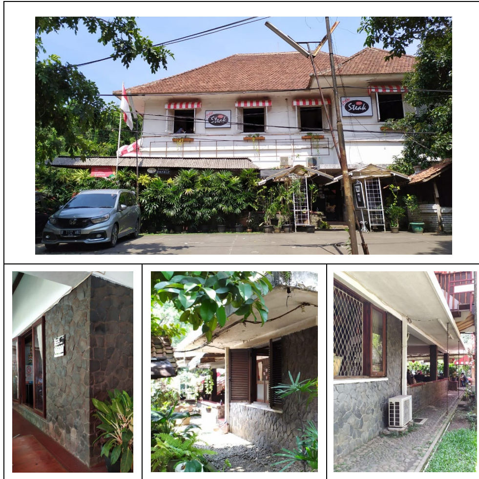
Figure 5. Architecture of Rumah Macaroni Panggang and Stone Wall Finishes Source: Private collection
