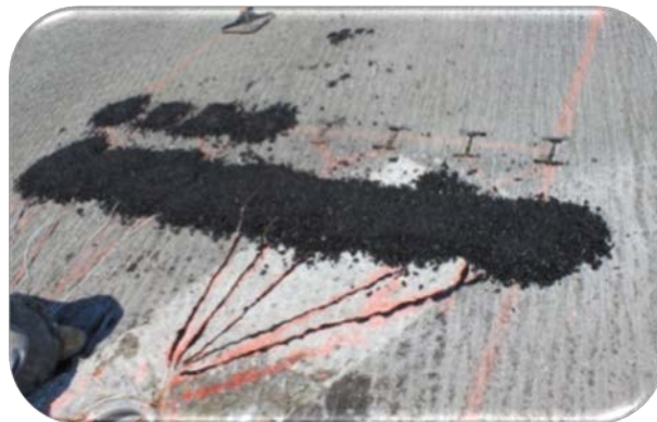
Figure 7. ASG installation at Newark Airport
