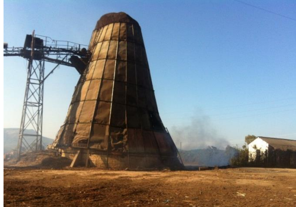
Figure 2 Incinerator at the Pine Company.
