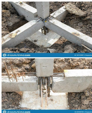
Figure 5. Precast joint placement
