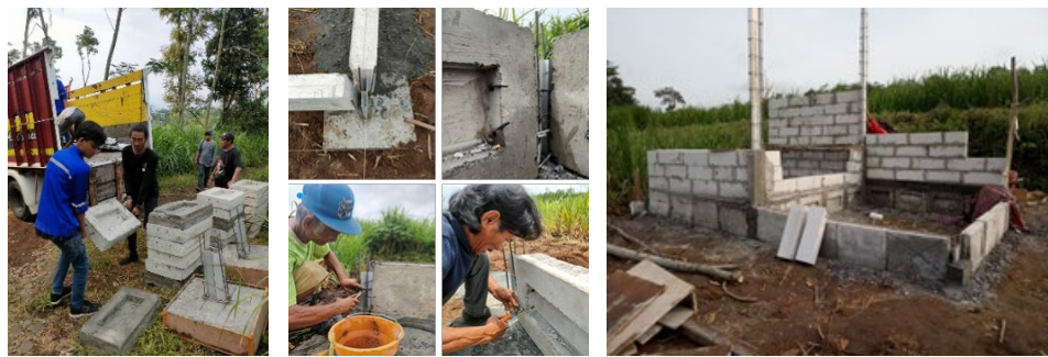
Figure 11. Implementation of the Concrete Puzzle Panel Prototype
