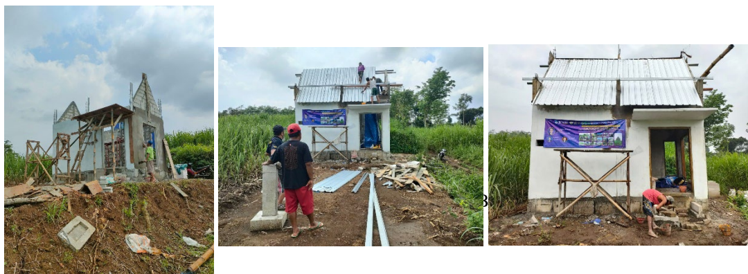
Figure 12. Implementation of the Concrete Puzzle Panel Prototype
