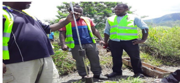
Figure 7. Dynamic cone penetration test (DCPT) on Erap Bridge site
