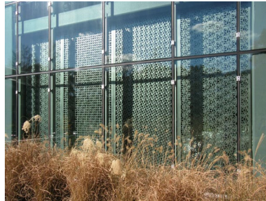
Figure 3. Tessellate: Using four basic geometries: hexagons, circles, squares and triangles Source: Simons Center | Zahner — Innovation and Collaboration to Achieve the Incredible 2016
