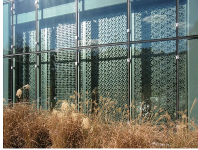
Figure 3. Tessellate: Using four basic geometries: hexagons, circles, squares and triangles Source: Simons Center | Zahner — Innovation and Collaboration to Achieve the Incredible 2016
