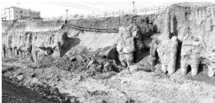
Figure 4. Basement perimeter surrounded by shoring piles (Zumrawi et al., 2016).
