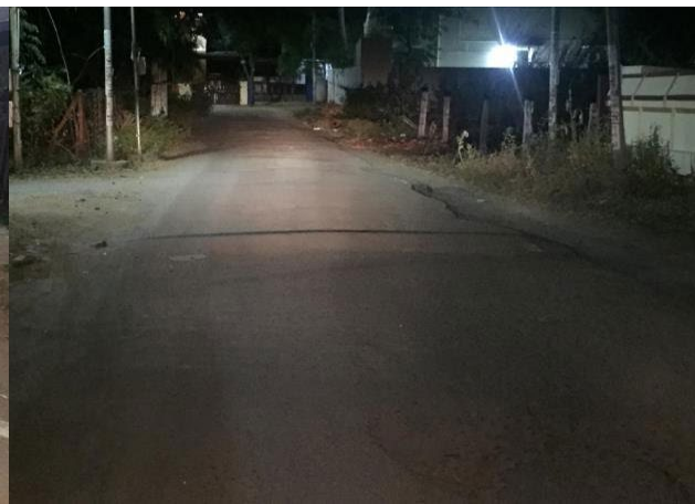
b. Hump in urban area without markings
