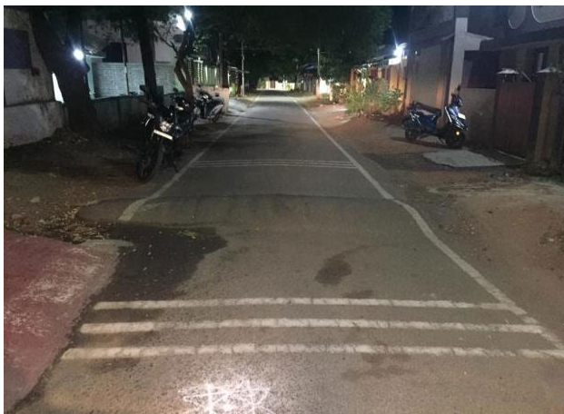
Figure 3 a. Hump in urban area with markings
