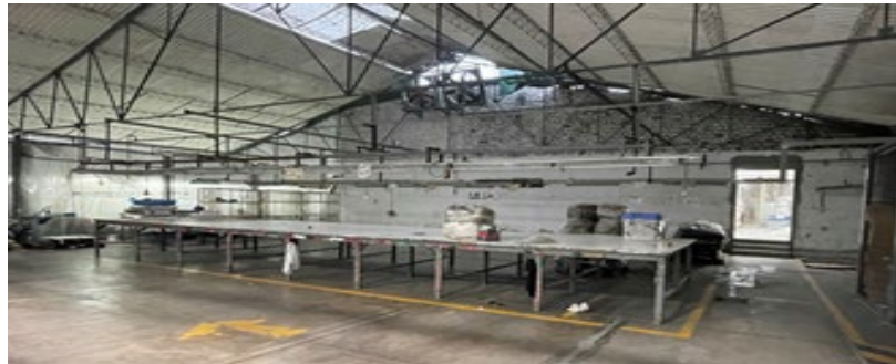
Figure 12. Luminaires at the workstation before the redesign
