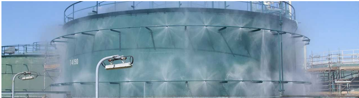
Figure 3. External Sprinkler system
