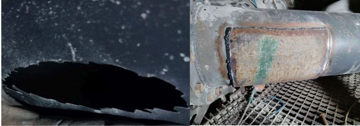
Figure 14. Whole on pipeline and repair
