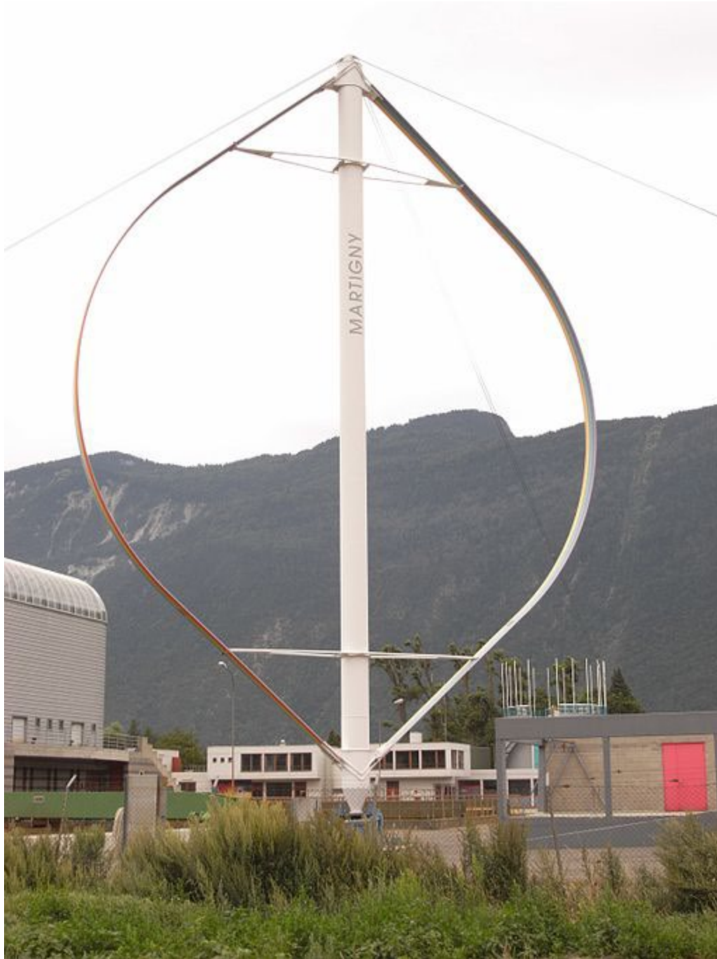
Figure 4. Darrieus vertical-axis wind turbine in Martigny, Switzerland
