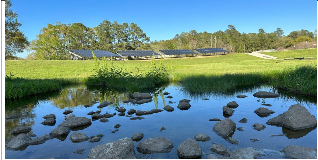
Figure 3. Fully constructed solar array of 80 x 420W PV panels on campus
