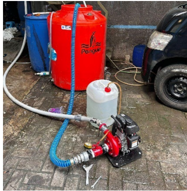
Figure 6. Installation of Flame Freeze Connector with Pump and Suction Hose
