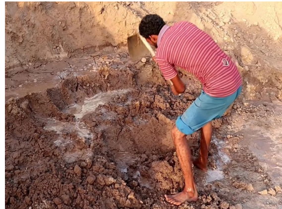
Figure 7(b) : Clay mixing process.
