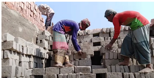
Figure 7(e) :Brick loading Process .
