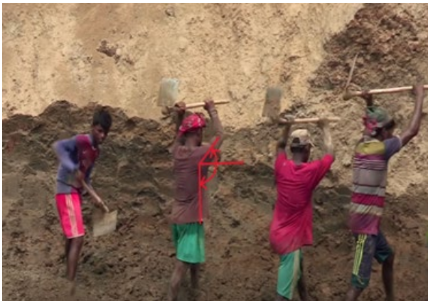
Figure 7(a) : Digging process.
