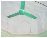
Figure 47. Application of electric fan inside the dome (Hossain 2006)
