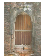
Figure 46. Window from outside
