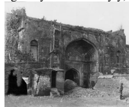
Figure 8. South wing from courtyard in 1950 A. D
