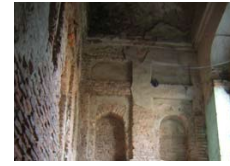
Figure 37. The original plaster has been removed inner wall (Source: Author 2018)
