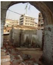
Figure 23. Razing wall By Madrasa (Mowla and Shaikh 2013)
