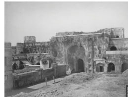
Figure 5. South Wing from the Court Yard in 1870 A.D.
