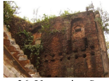
Figure 36. Vegetation Southern gate (Source: author 2010)
