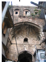
Figure 17. Southern gateway of Bara Katra views from the riverside (Source: Author 2018)
