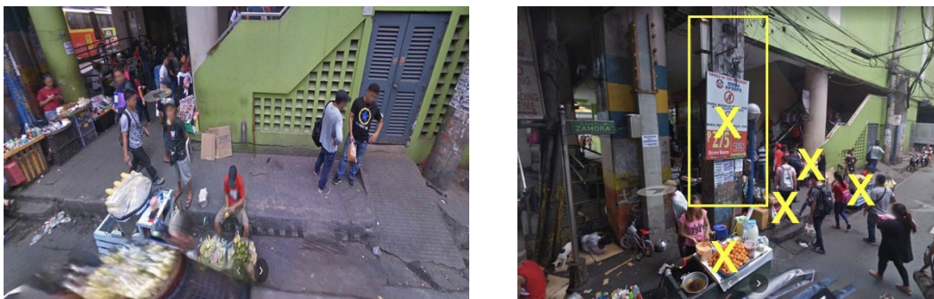
Figure 4. (From left to right) Lack of facility features that aid PWDs and elderlies. Accesses are obstructed by vendors and their merchandise
