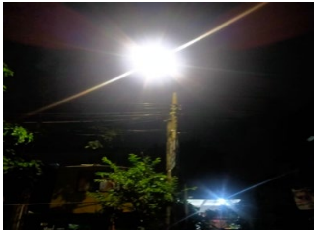
Figure 1. Standard Automatic Streetlight
