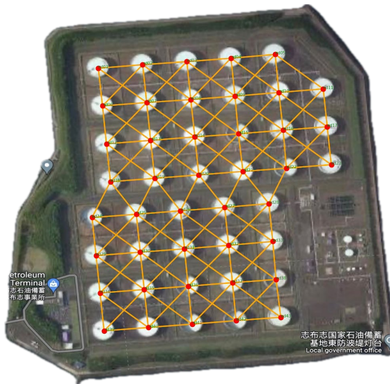
Figure 3. The Satellite photo of the plant to identify the location of each node
