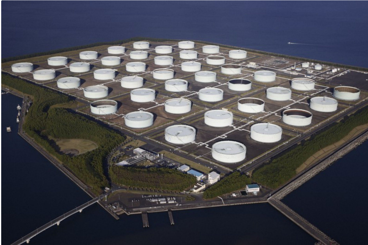
Figure 2. The aerial photo of the Shibushi national petroleum stockpiling base in Kagoshima Prefecture. (Mainichi).
