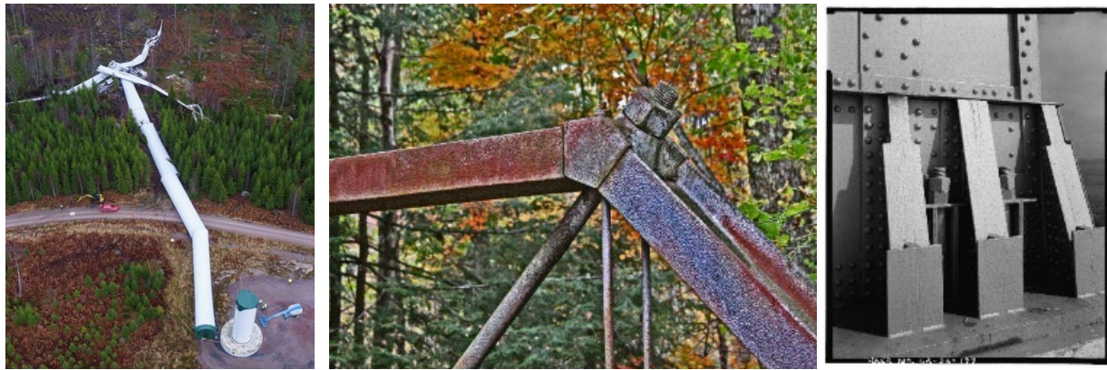
Figure 1. A wind turbine structure that collapsed due to a bolt failure (Swedish Accident Investigation Authority, 2017), picture is obtained with permission from Vestas Wind Systems A/S, Sweden (Left). Bolted bridge structure in Ohio (Center). Bolts at the base of the pier W-6 tower of the San Francisco Bay Bridge (Right). (Center and Right pictures are in the public domain, source: Wikimedia Commons).
