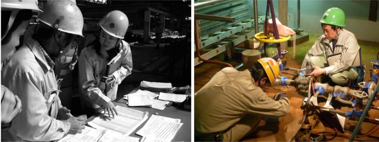
Figure2: Observation at Power Plant Manufacturing and Construction Sites
