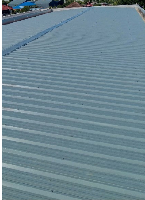
Figure 2. Site photograph of the case study building's rooftop area in Bangkok.
