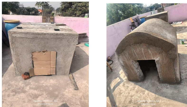
Figure 2. On Site images of two rooms with flat and inverted U shaped roof
