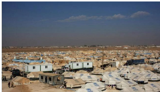
Figure 2. A picture of the modular, caravan-based structures in the Za'atari Camp (Carlisle, 2022) These structures demonstrate how extreme weather conditions, including heat and rainfall, contribute to material degradation over time.
