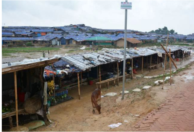
Figure 3. A picture of the temporary shelters at Cox's Bazar, constructed with bamboo and plastic sheeting (Shohag, 2023).
