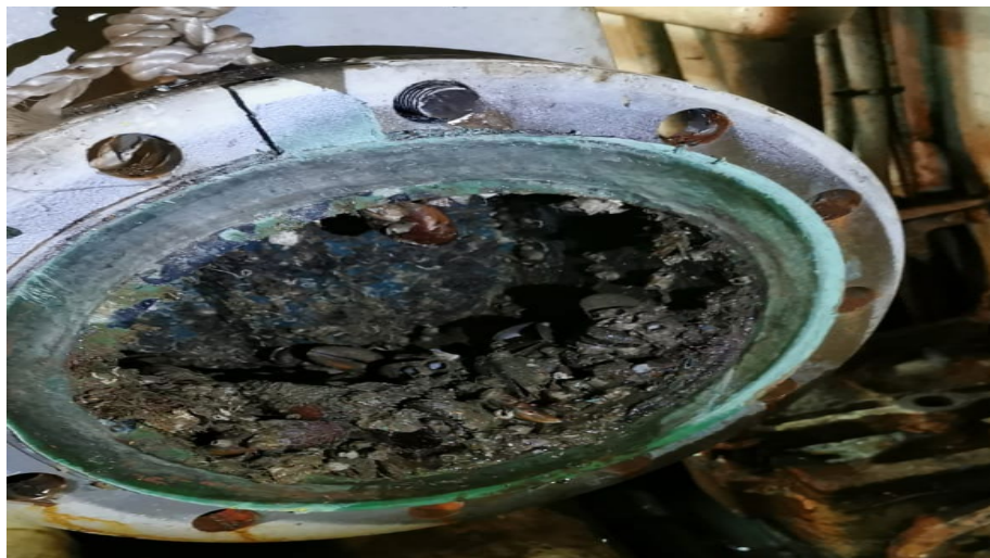
Figure 7. Condenser Pipe Blockage Due to Sea Growth.
