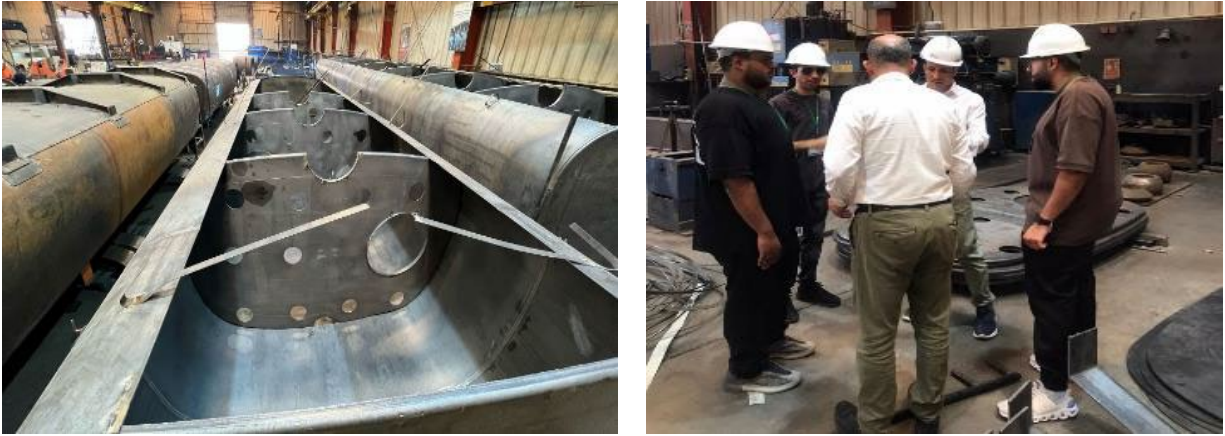
Figure 8: Manufacturing process for the oil tanks, The Mula company in Kuwait
